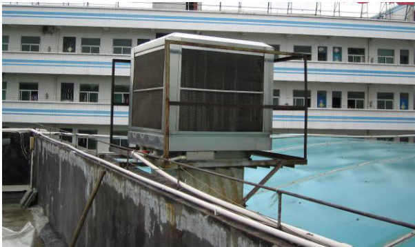
Fresh Air Intake for the Office
