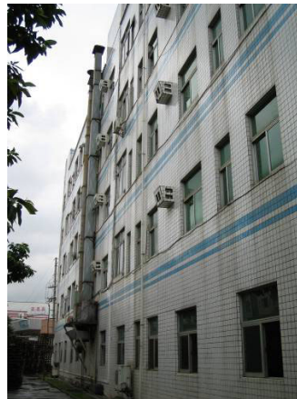
Separate Stacks for Cooking Fume and Exhaust from the Diesel-fired Stove from the
