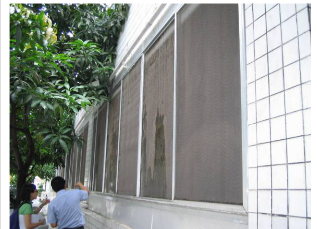
Water-cooled Screen for the Production Workshop
