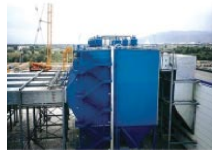
Example of an electrostatic precipitator in a factory
